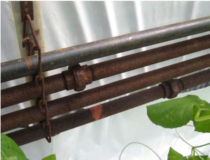
New pipe replacement, example for leakage avoidance
