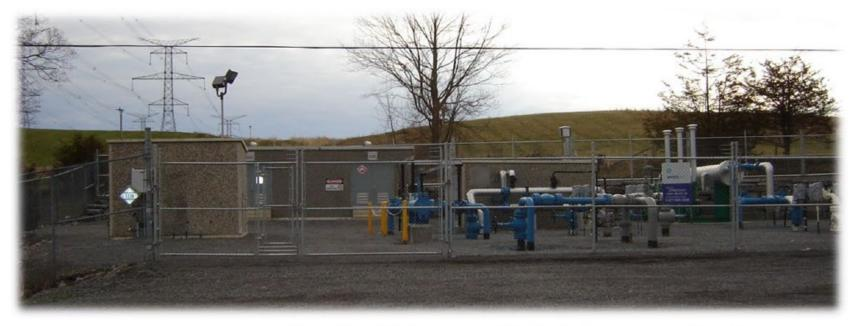
Transition inlet pressure (1000psi) then a reduced outlet pressure
