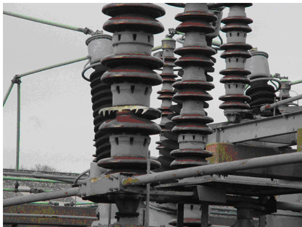
Figure 11: Cracked Insulator Porcelain – 3 rd from Bottom
