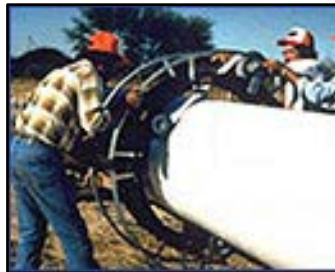
Tape coat and tape wrap
