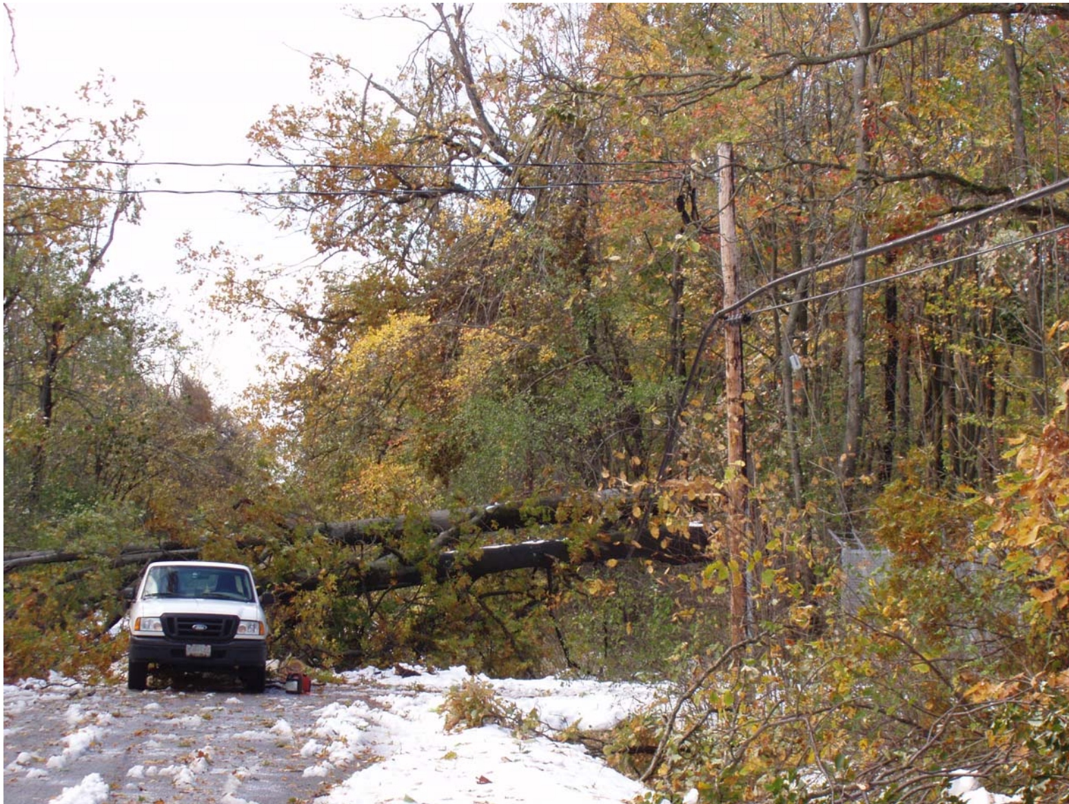
Large trees bring down power lines located on the opposite side of right-of-way.
