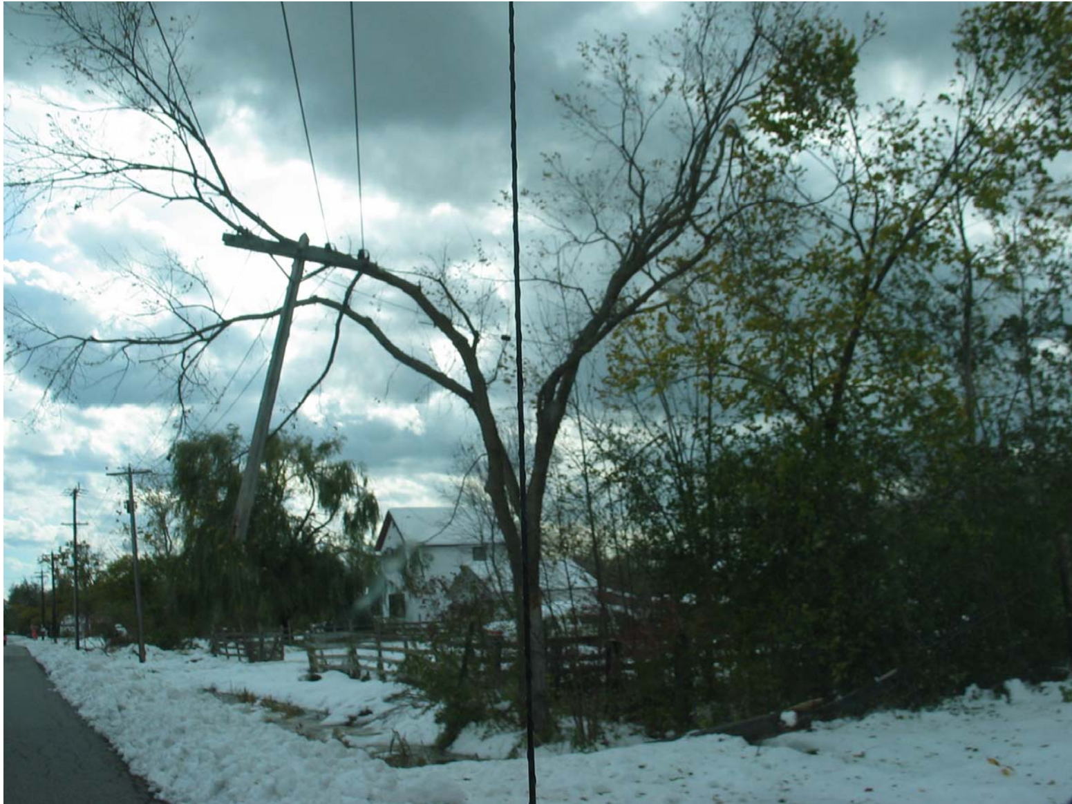
Poles shear from loading of snow, wind and trees.
