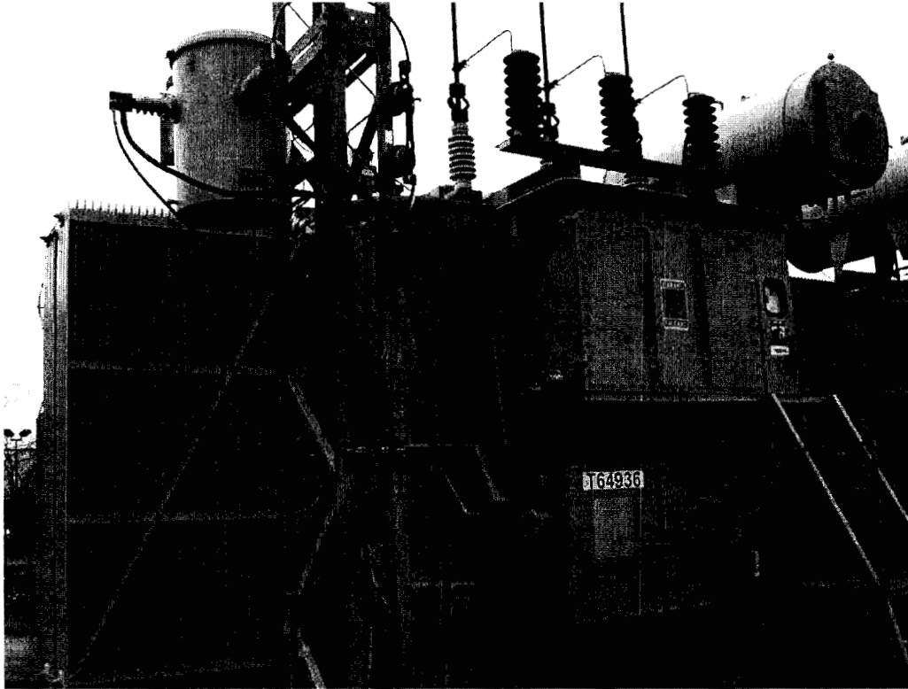
Well Maintained Older Transformer
