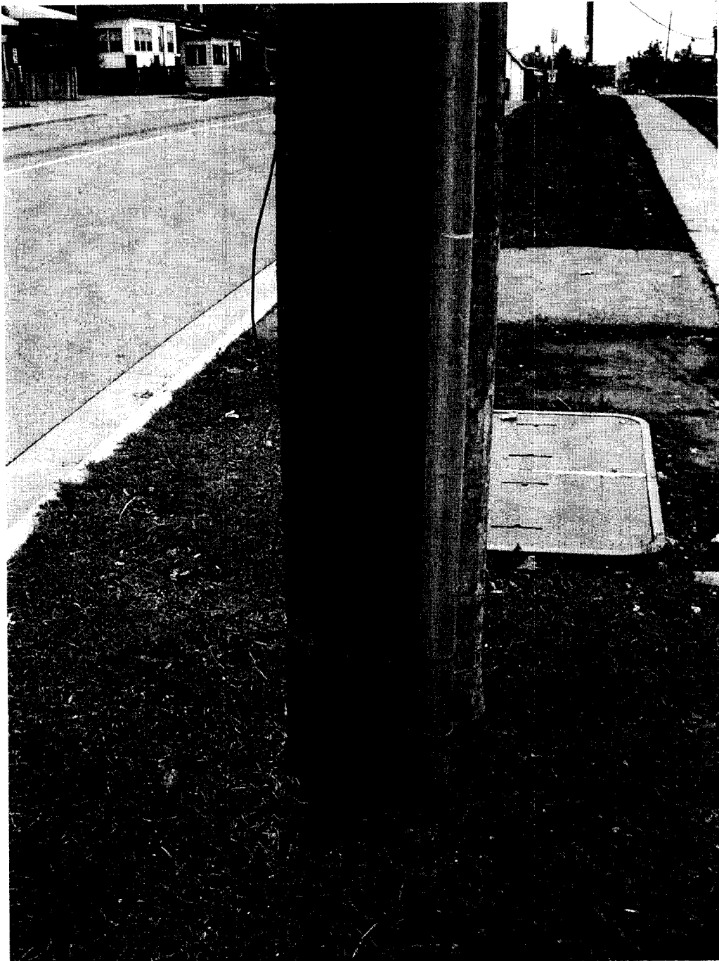
Exposed Ground Lead
