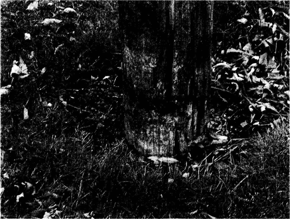
Pole Rotting at Base
