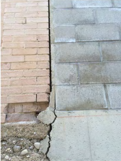
-Building structural condition?
